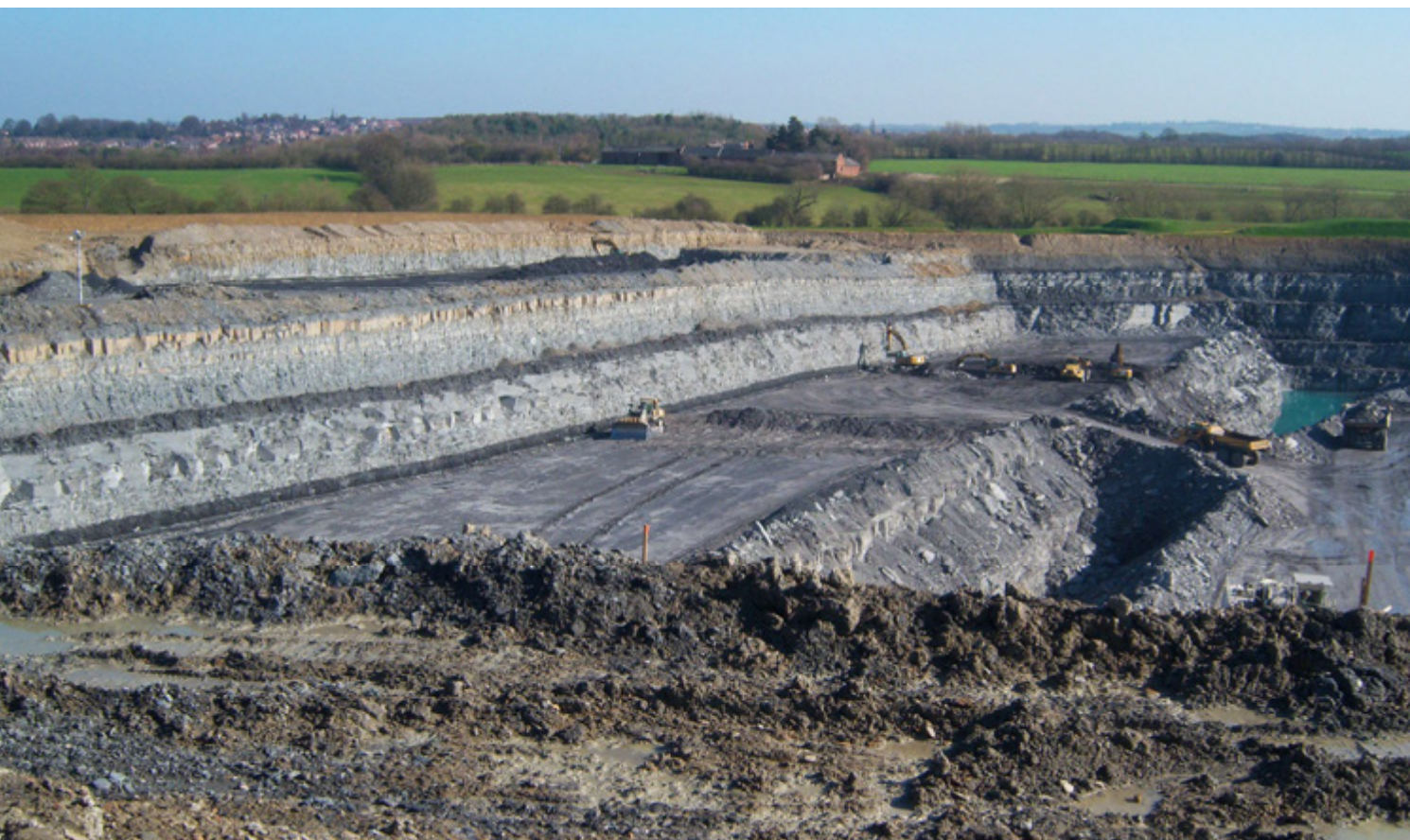
Lodge House - pre soil replacement 2011
