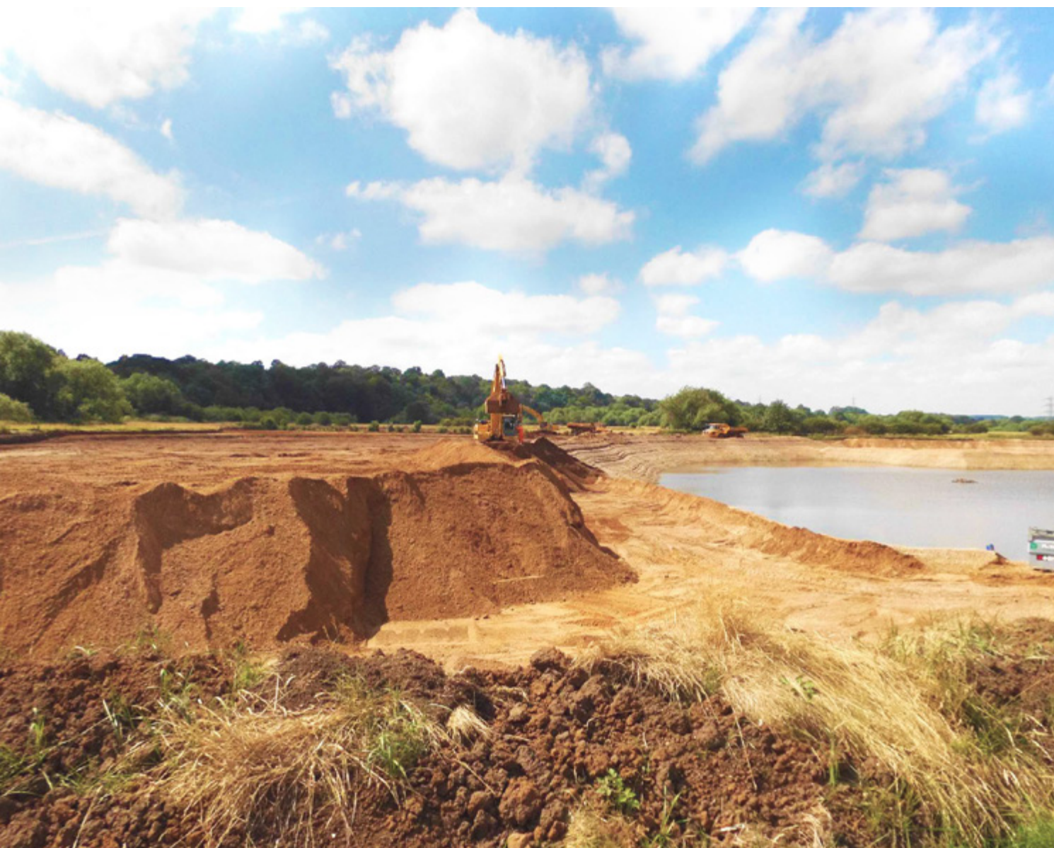
Shardlow Quarry - sand and gravel extraction
